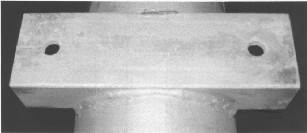
Pic 01 Tower locking plate, rear of pole
